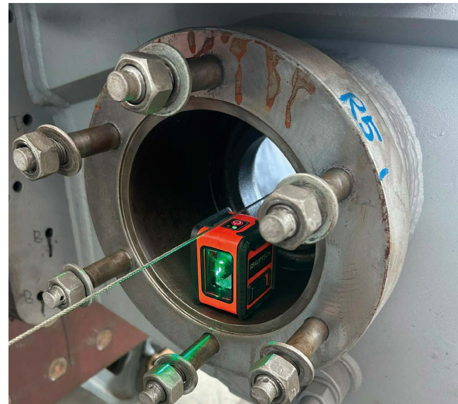
With the cylinder block in place work can start on final alignment of the valve gear.
