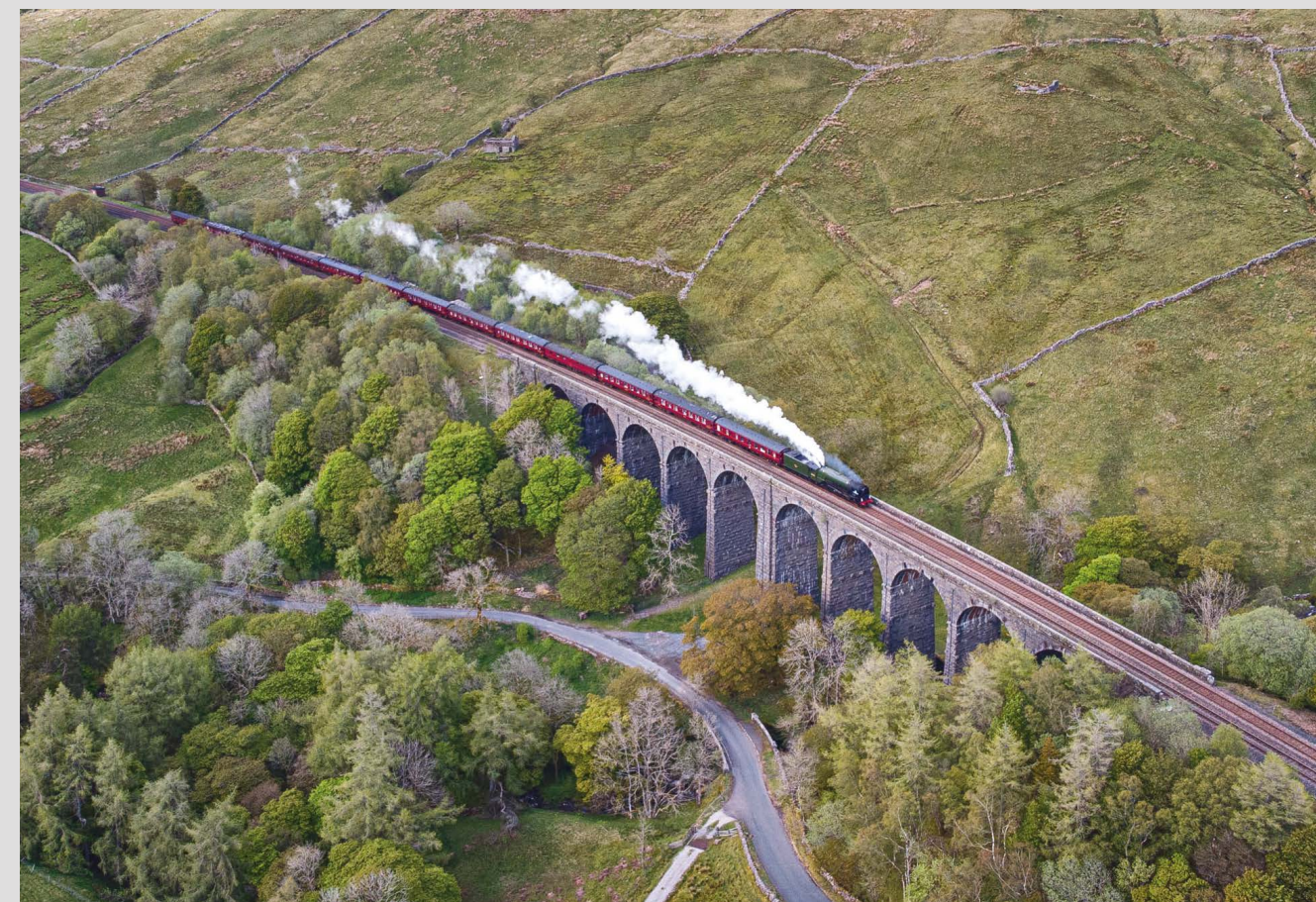
Tornado crosses Dent Head Viaduct with 'The Pennine Explorer' on 22 nd May 2021.
